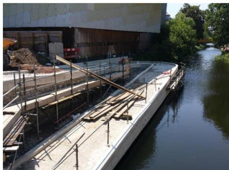
Works have been going on to construct a brand new pedestrian and cycle bridge, uniting the two sides of the canal path, and the reflection of the gabion walls and polished steel railings on the water show a project excitingly close to completion. Just the connecting section remains to be built.
