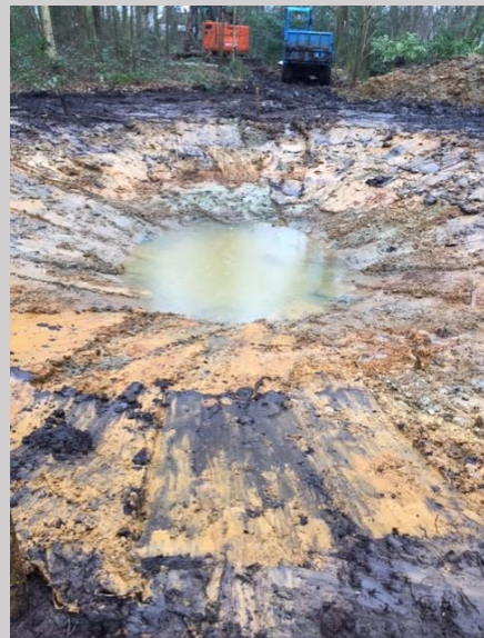
Photograph 4. SWC8 construction of pond January 2020.
