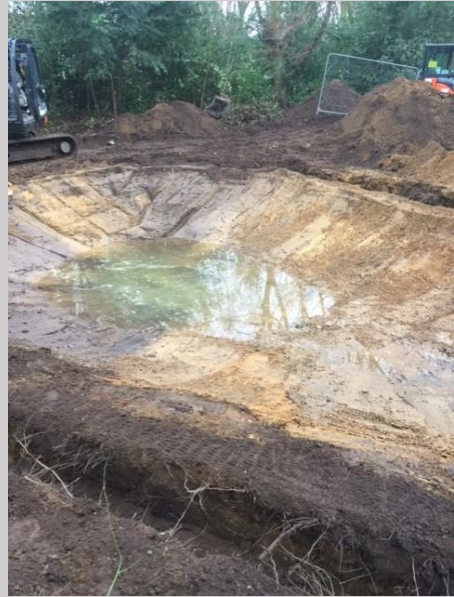
Photograph 2. CWC2 pond construction in January 2020.
